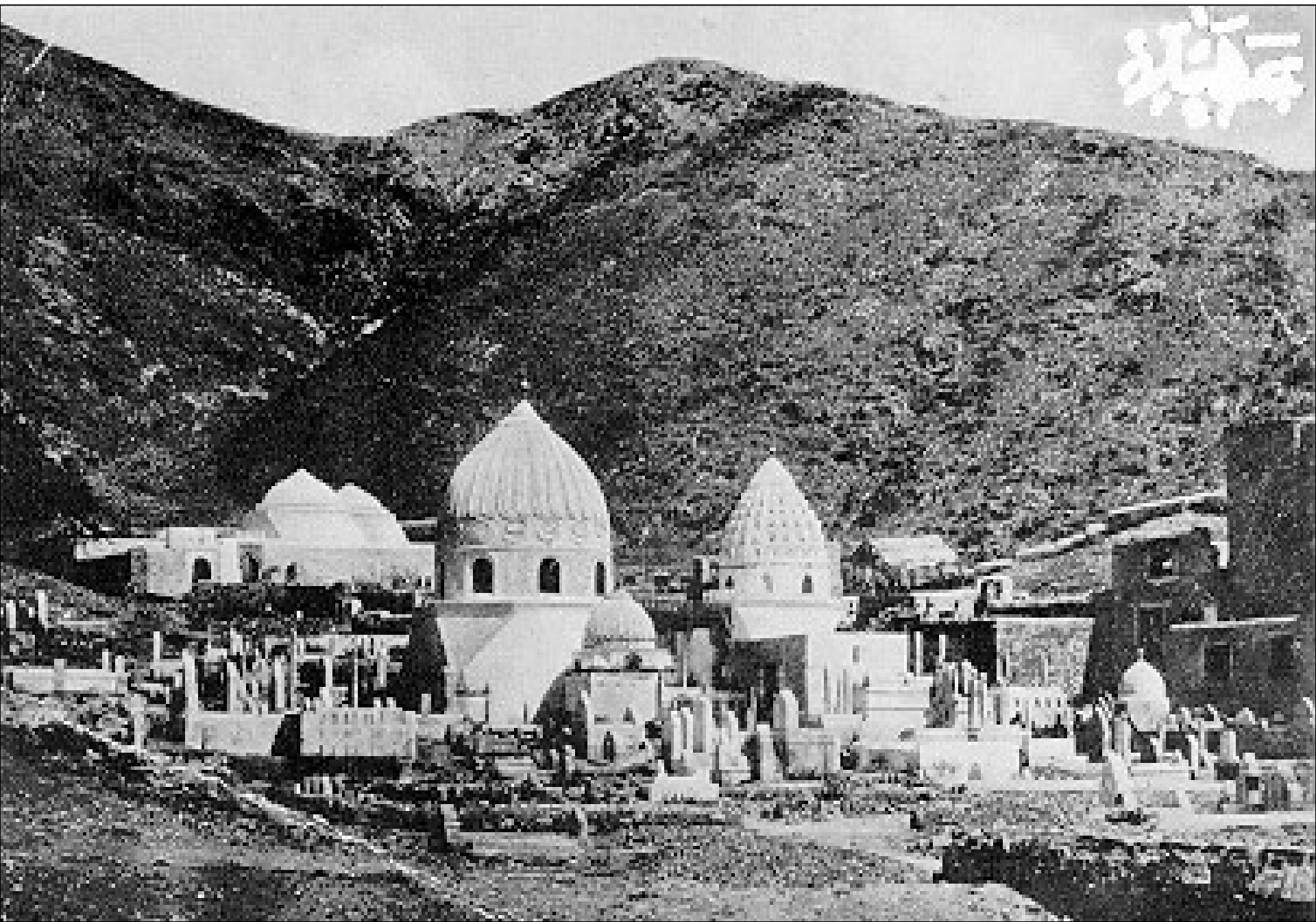
Jannat ul Moala, before destructions – Macca.
